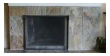
One rule of thumb on cutting tiles – try not to leave less than ½ of a tile remaining. If you need to cut 2/3 of a tile off, try cutting half of that amount off of two tiles instead. This has particular application when filling the space between the pilasters and the firebox. However, with exceptionally large tiles, you may need to take off more than ½ as shown in the fireplace above.
